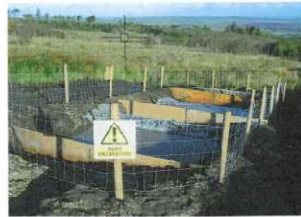
COMPLETED SETTLEMENT POND SYSTEM
